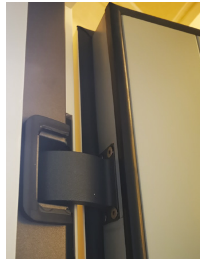
Dettaglio cerniere e braghettoni completamente in legno Detail hinges and braghettoni completely in wood
