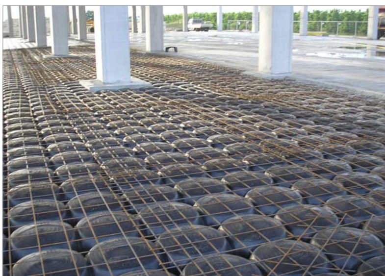
Cella frigo negativa - Alfonsine (RA)
