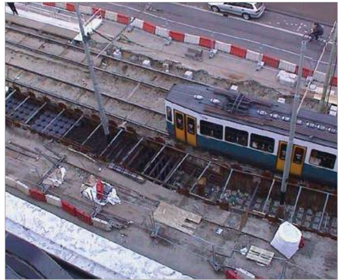
Renovation of a train platform
