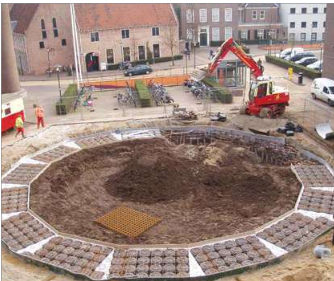
Tree root protection (Waterblock Holland)
