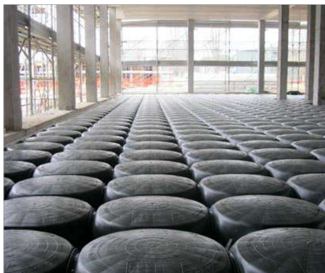
Building for sanitary use
