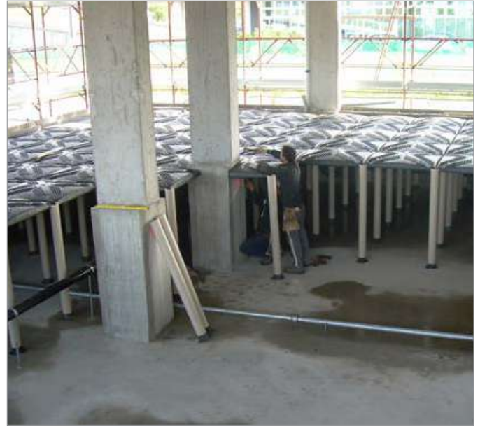
Building for industrial use
