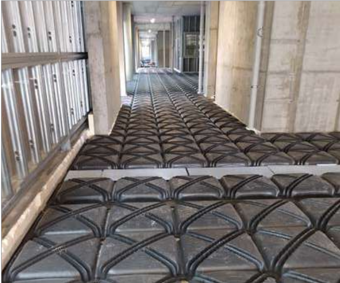
Building for industrial use
