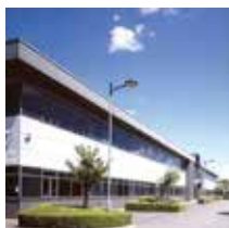
Redhill Data Centre, Redhill, Great Britain.
