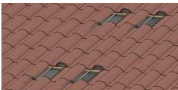
2.9. Fasten the structure to the 4 perforated steel strips (10) using 4 bolts, 4 nuts and 4 washers
