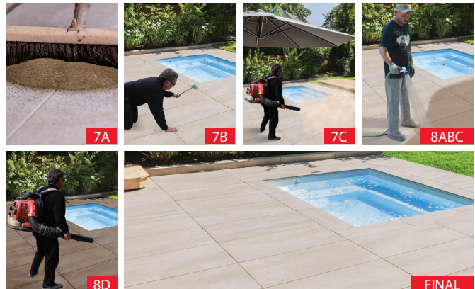
GATOR TILE SAND INSTALLATION STEPS
